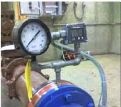
The One Series mounted on an isolation ring for monitoring wastewater.
