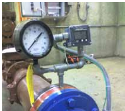
The One Series mounted on an isolation ring for monitoring wastewater.
